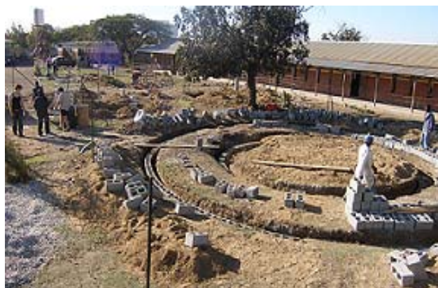
Construction of 1 st Library, Lusaka, Zambia. Completion Date: November 2006
