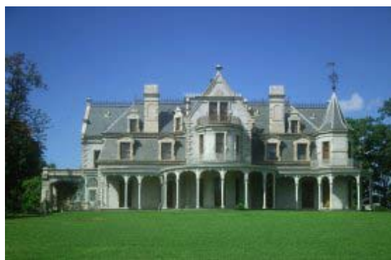
The Museum is one of the earliest Second Empire Style country houses built in the United States, and one of the finest surviving structures of its kind.
