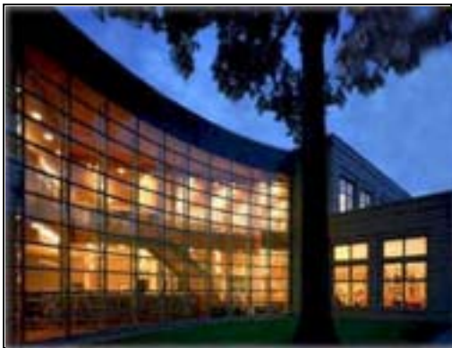
An outside view of the Peterson Wing at the Greenwich Library.
